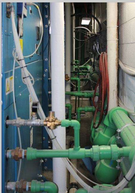
In the Sheraton Nashville Downtown hotel's laundry facility, 4-inch main headers (hot and cold water) run along an exterior wall, with Aquatherm fusion outlets bored through them to feed each washer. With more than 400 valves and fittings, the PP-R pipe can typically transition to nearly any fixture.
