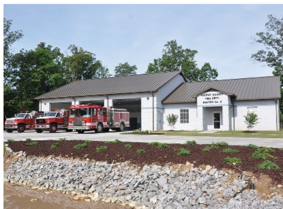
Benefits of metal roofing include excellent hail and load resistance, high recycled content, long service life, and low maintenance costs.
