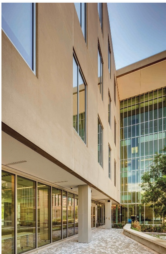
Precast panels were ideal for the tight project site on Canal Street in New Orleans' downtown core, which limited crane access. At only 28 pounds/sq. ft., compared with 78 pounds for conventional precast panels, a smaller crane could be used.
