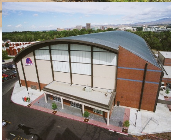
The Caven-Williams Sports Complex at Boise State University, Boise, ID, demonstrates how curved metal roofing and its shape blends well with the mountainous terrain. MBCI's BattenLok standing-seam roof panel, with its classic pan profile and pencil ribs, installs easily on a curve.
