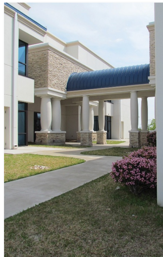
Metal roofing is ideally suited to curved roofing. Because steel can be rolled very thin, it can go over curved surfaces without special forming or stressing.
