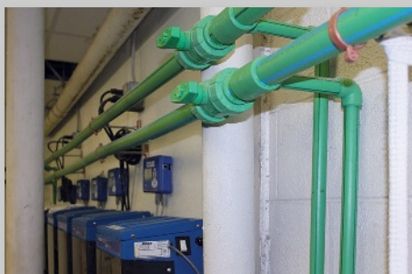
One benefit of using Aquatherm PP-R pipe in the laundry facility is that the pipe has the ability to expand and contract more than metal pipe, so it is able to withstand the hydraulic force exerted on it by the valves in the commercial washers. Also, since the pipe has a natural R-value, even when 180-F fluid is flowing through it, it doesn't get hot to the touch.
